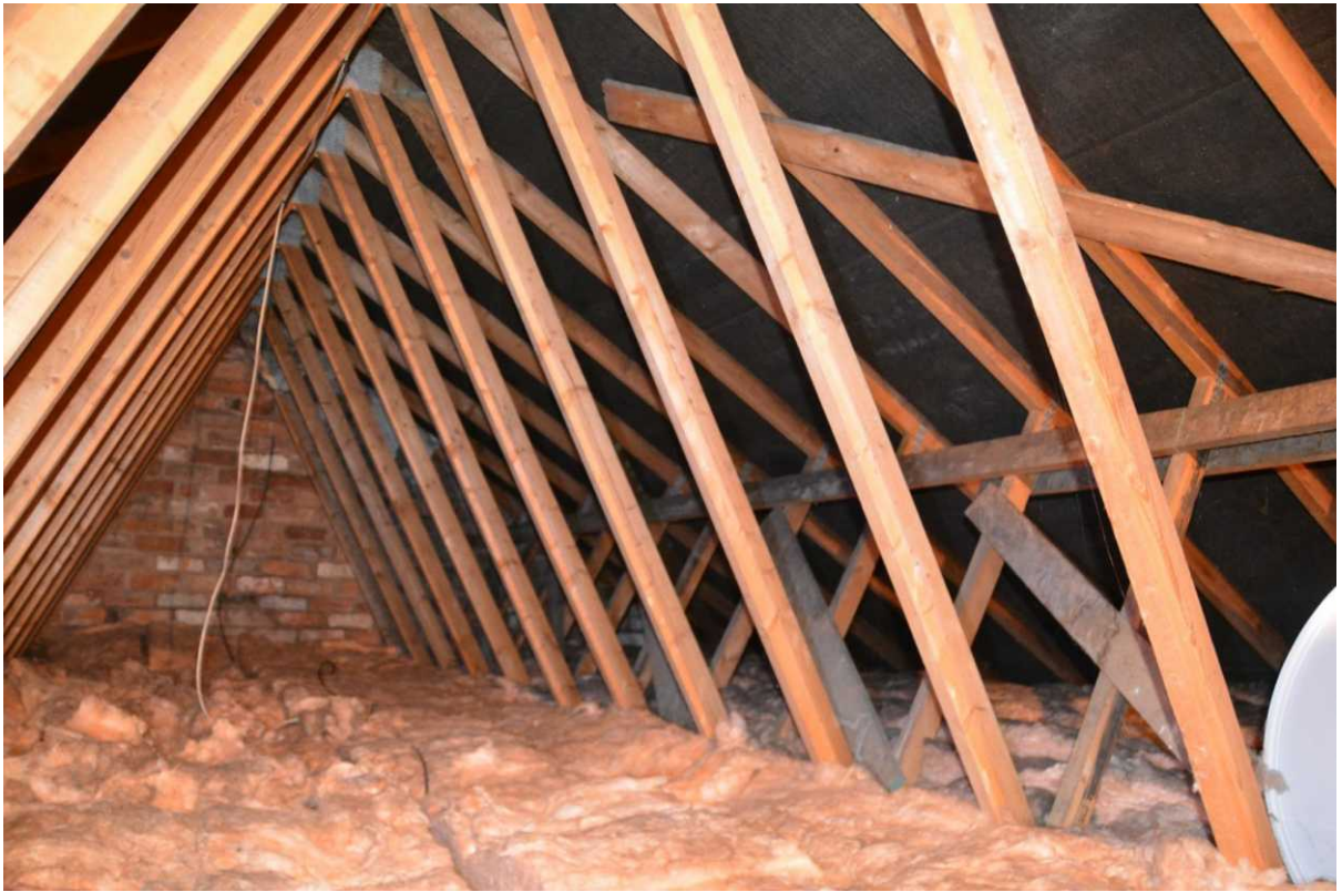
Trussed roof structure.
