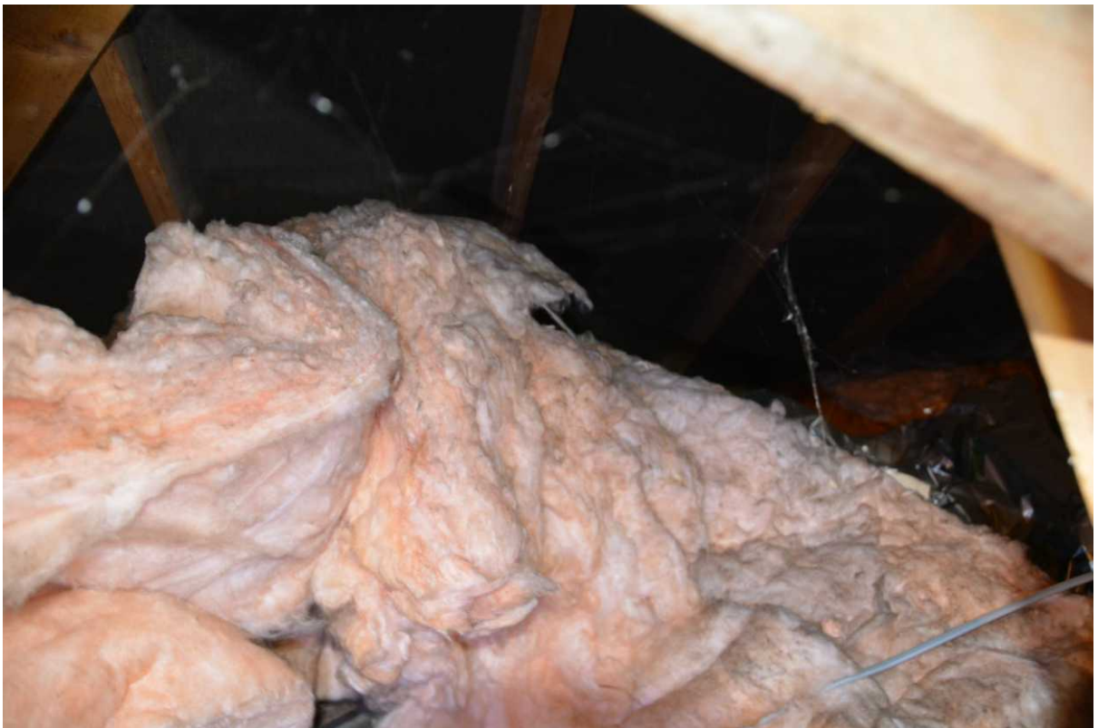
Wiring beneath insulation.
