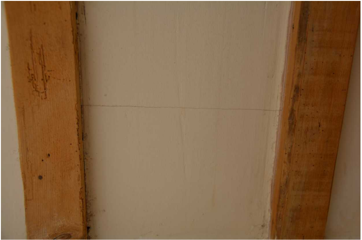
Shrinkage crack.
