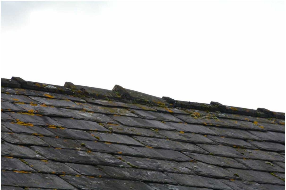
Moss present to ridge tiles.
