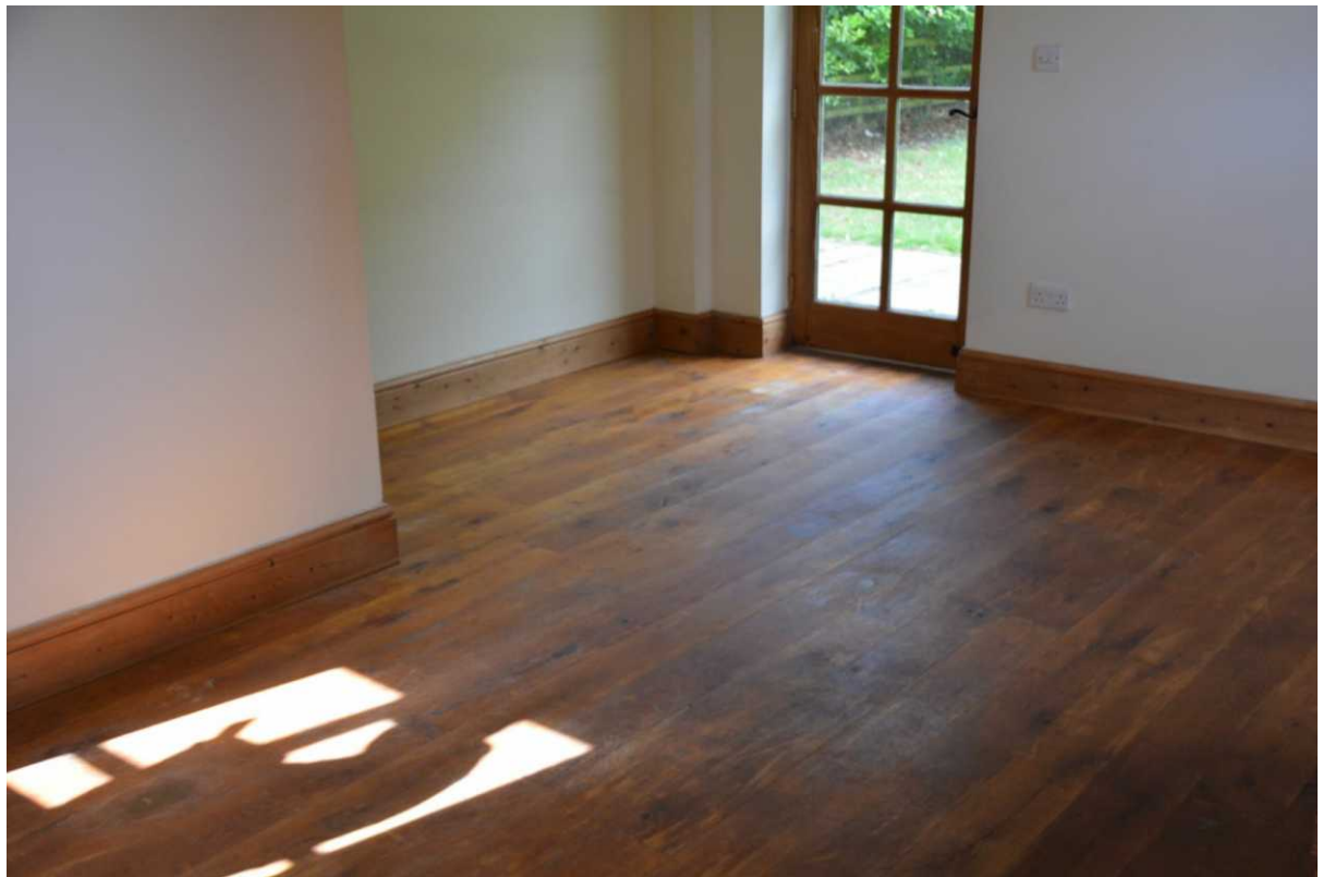
Floating timber floor.
