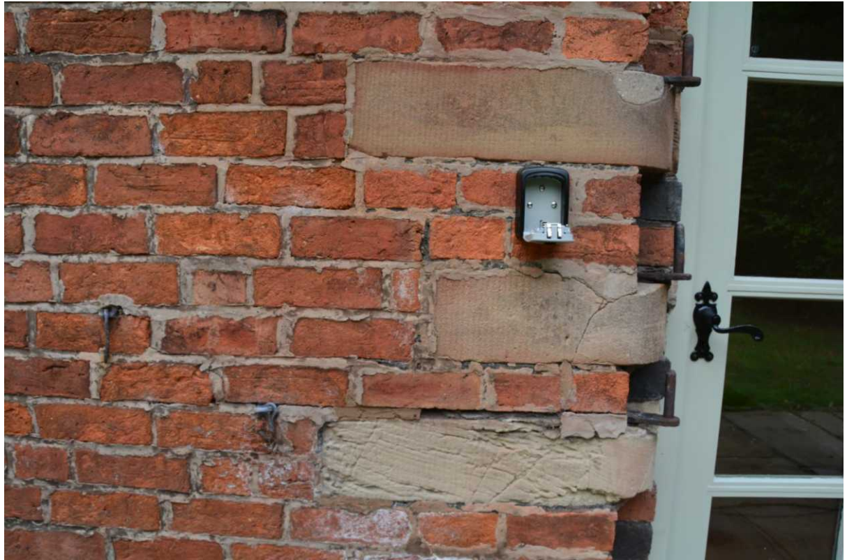
Sections of stone.
