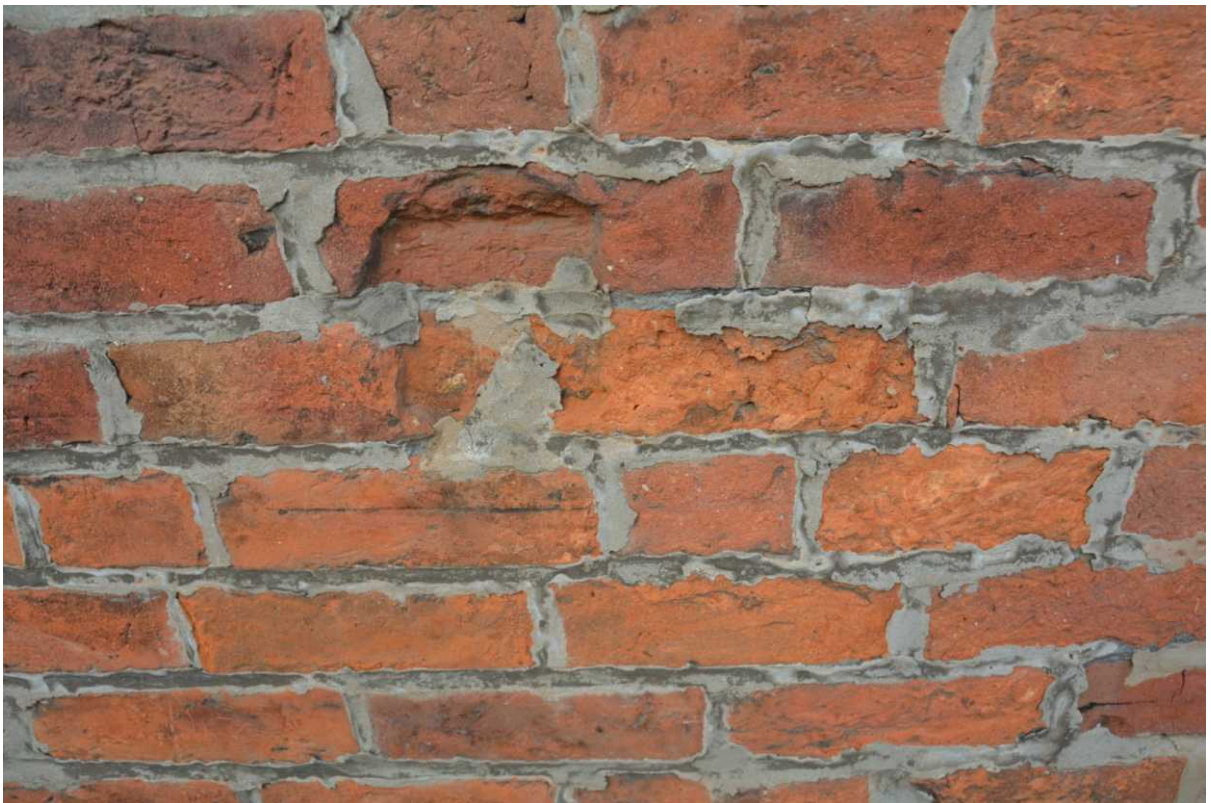
Spalled brickwork.
