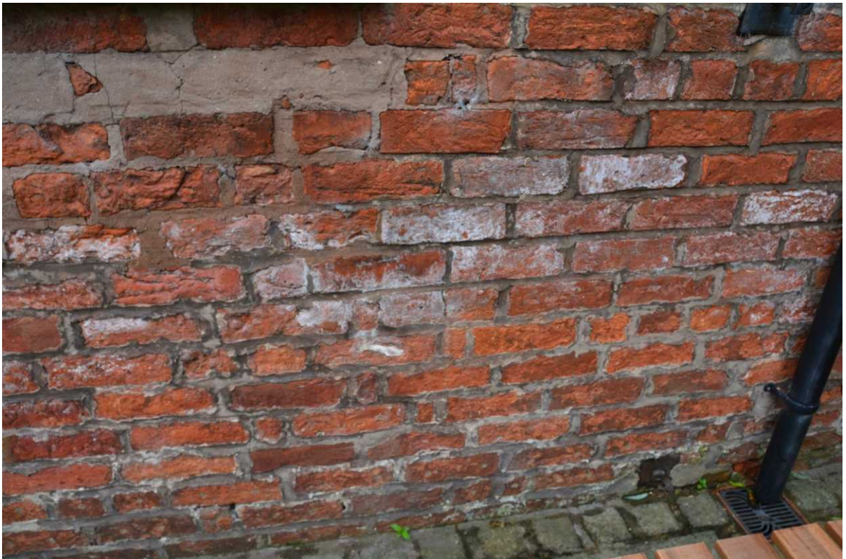
Efflorescence.
