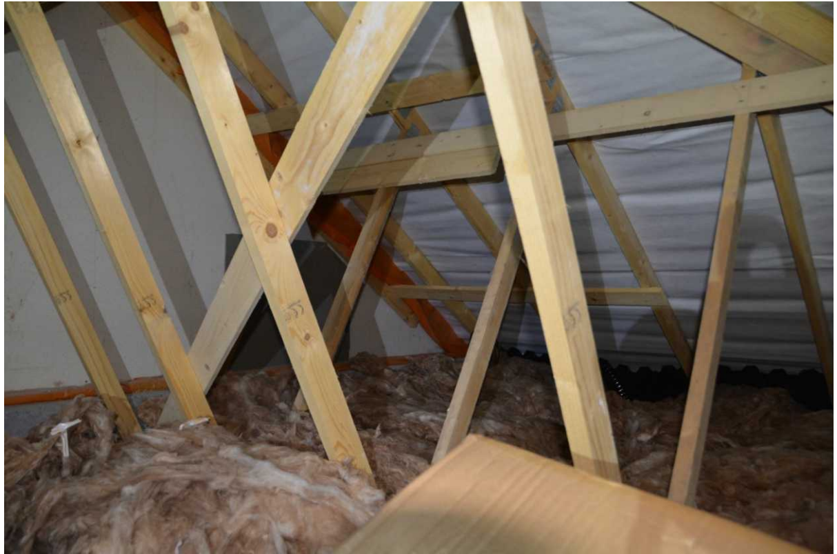
Trussed roof structure.
